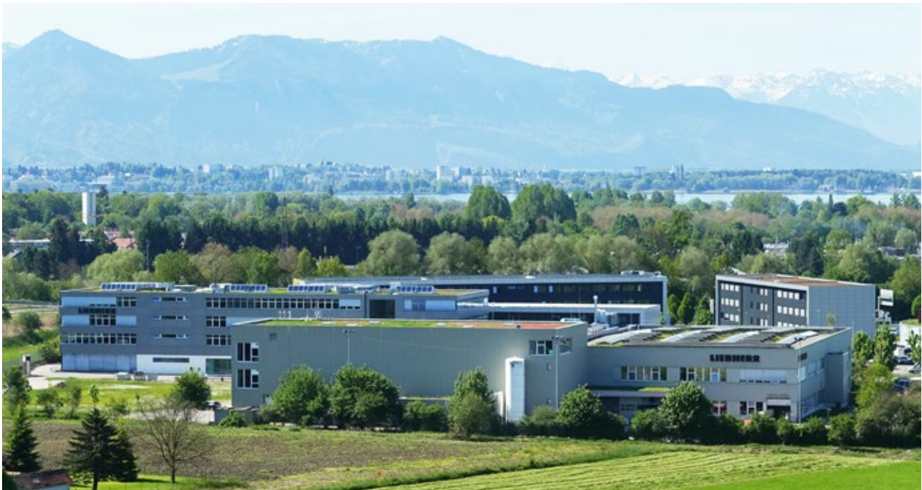
Liebherr-Elektronik GmbH, Lindau (Germany) – home of the aerospace electronics and industrial electronics business unit of the Liebherr Group
