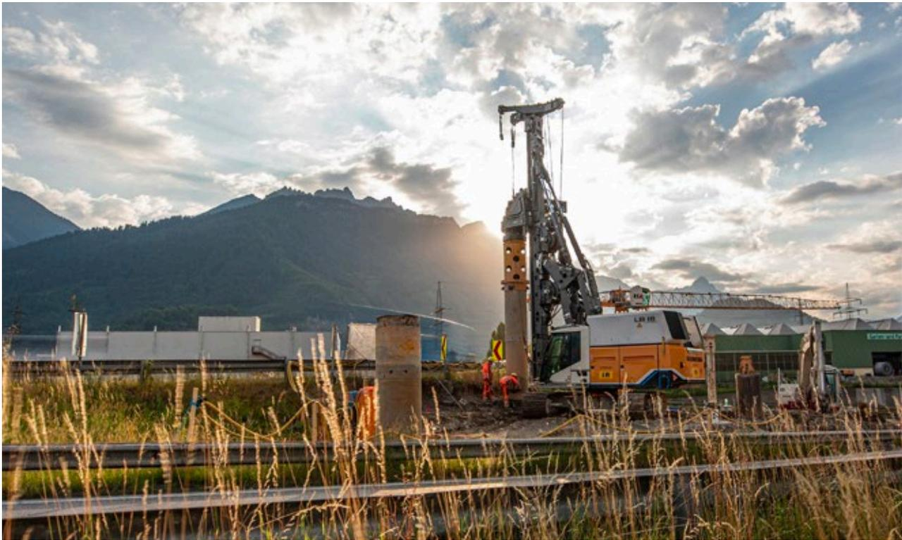
The first battery-powered drilling rig in the world, the LB 16 unplugged, is used on one of the largest roadwork sites in Western Austria
