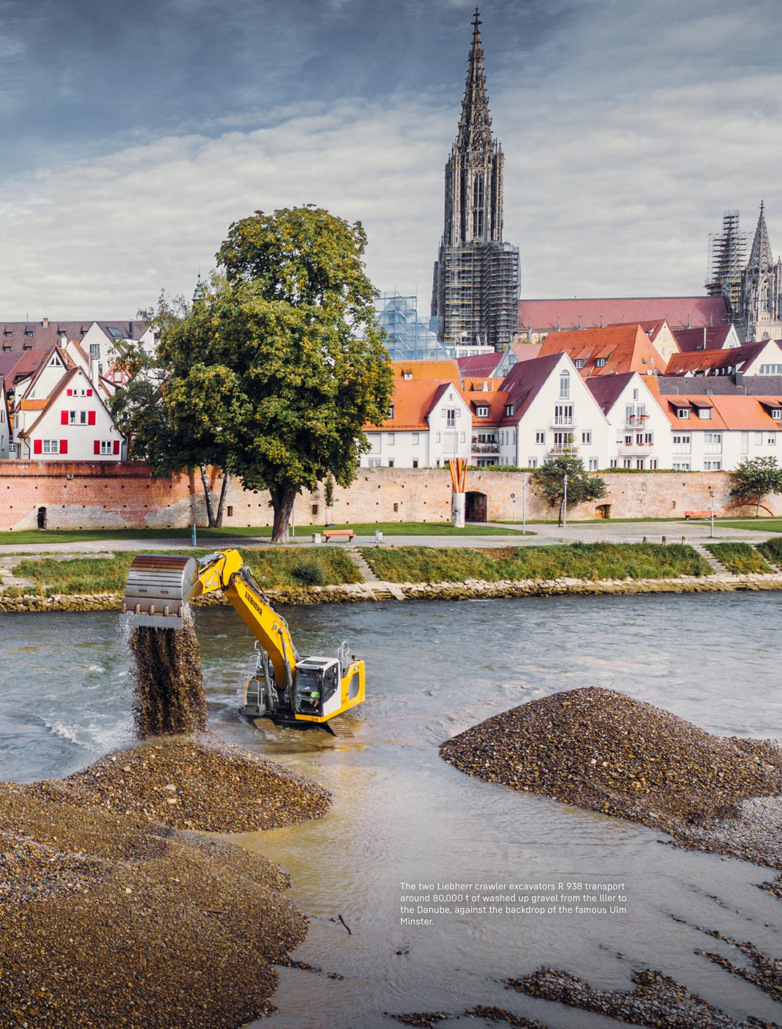
The two Liebherr crawler excavators R 938 transport around 80,000 t of washed up gravel from the Iller to the Danube, against the backdrop of the famous Ulm Minster.
