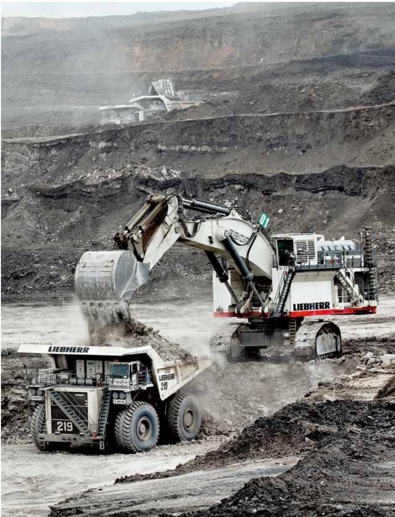
A well organised team: excavator and mining truck
