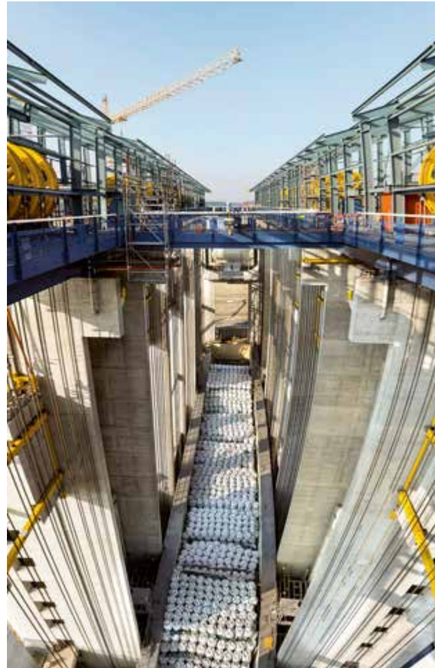
The ship lift's main axis
