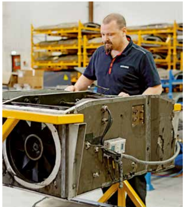
Inspection of an air conditioning system
