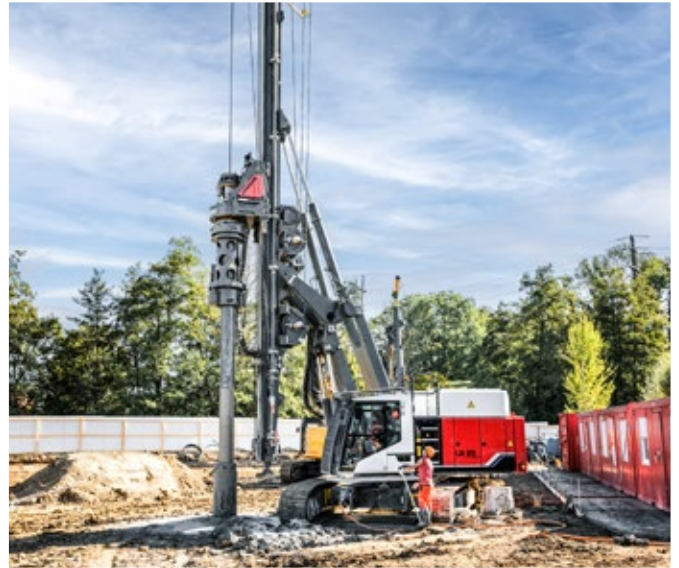
The LB 25 unplugged demonstrating its Kelly drilling capabilities in Zurich (Switzerland)
