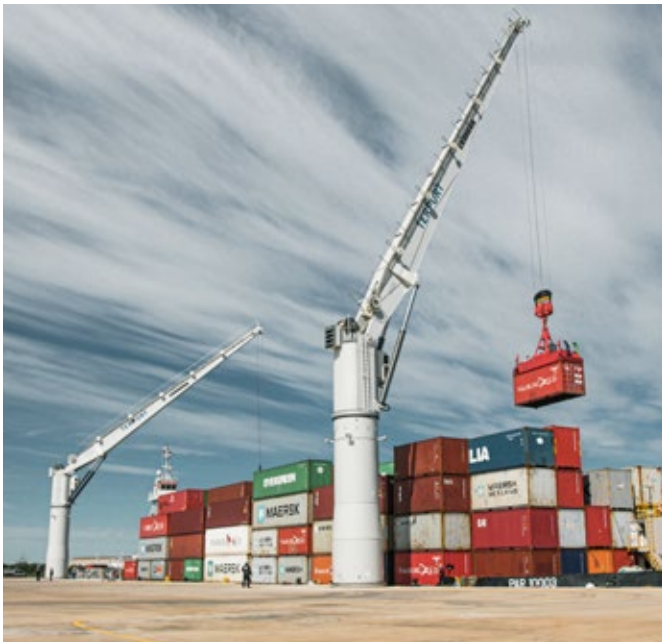
An FCC 280 fixed cargo crane handling containers in San Antonio (Paraguay)
