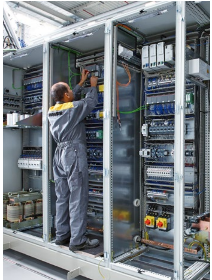
Installation of control cabinets for container cranes
