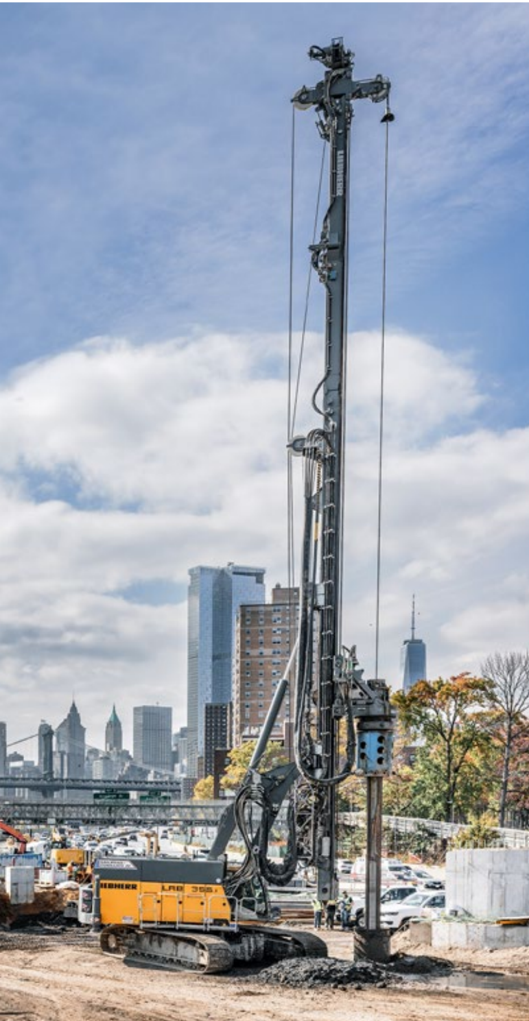
Kelly drilling with the piling and drilling rig LRB 355.1 in Manhattan, New York (USA)
