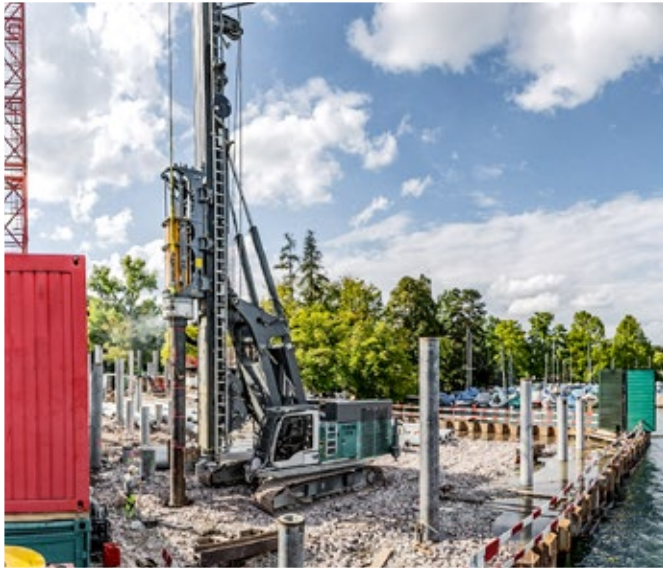
The LRB 355 driving spun piles with the hydraulic hammer H 15-10 at Lake Zurich (Switzerland)
