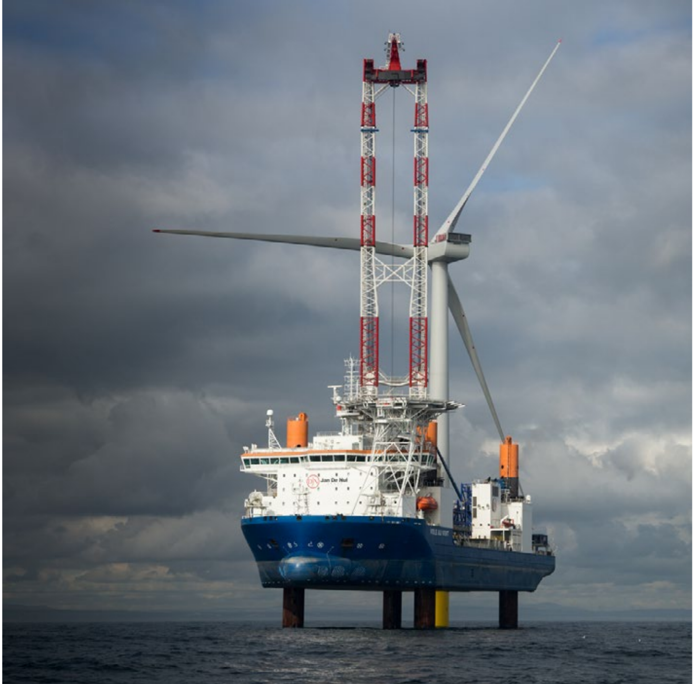
This CAL 45000 offshore crane, which is designed as a crane around the leg, in operation on-board the 'Vole au Vent', can lift up to 1,200 tonnes.
