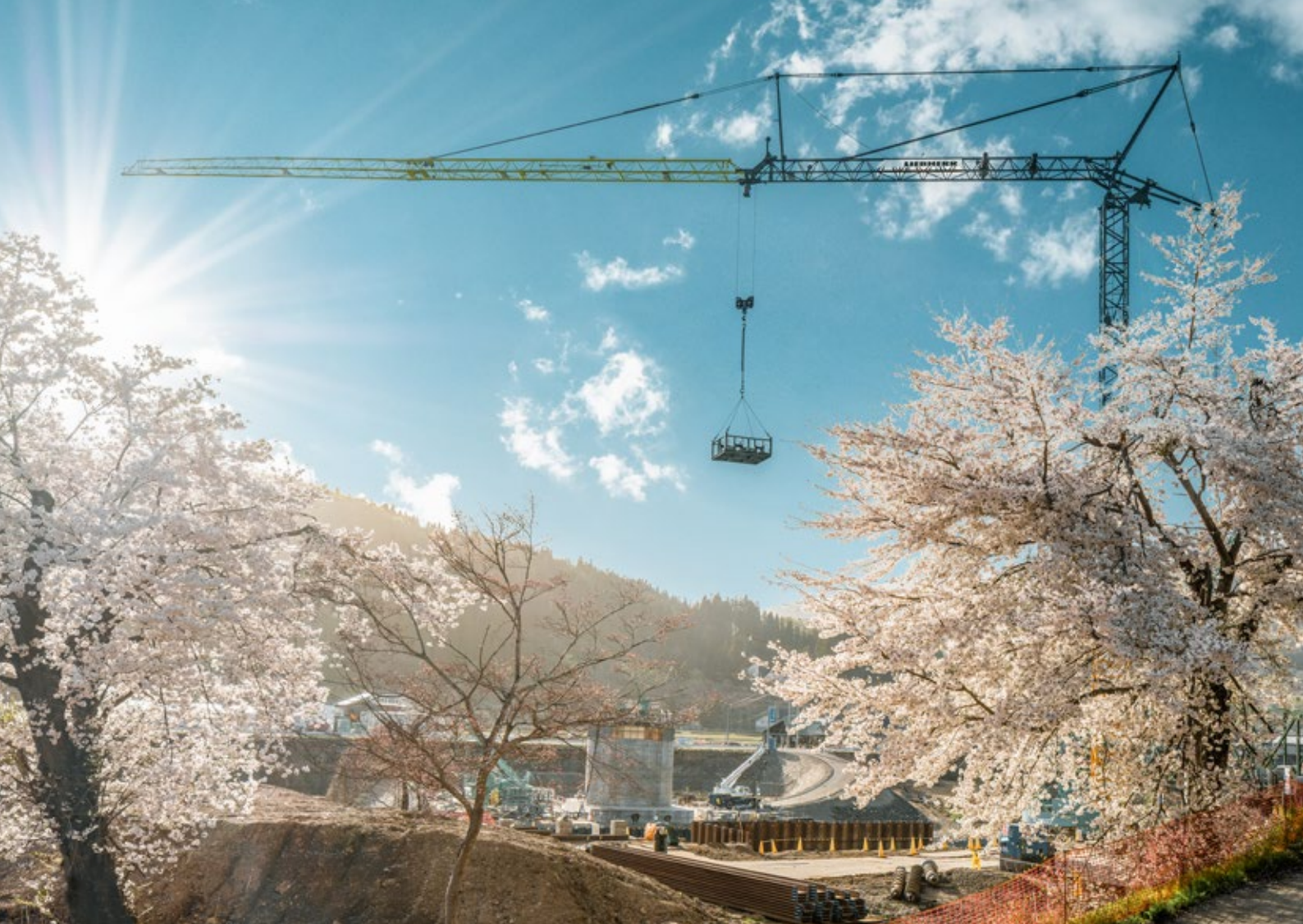
The 53 K fast-erecting crane at work on the construction of the YURII bridge in Nagano (Japan)
