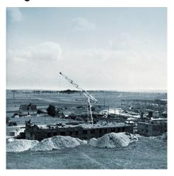
The TK 10 took two to three hours to assemble, compared to the usual cranes at that time, which took several days to erect.
