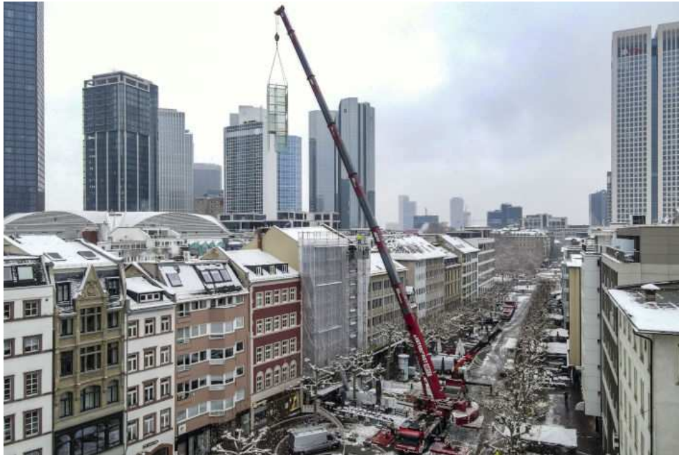
liebherr-ltm1230-5-1-adw-motive01.jpg Autodienst West installs an elevator shaft in Frankfurt city centre.
