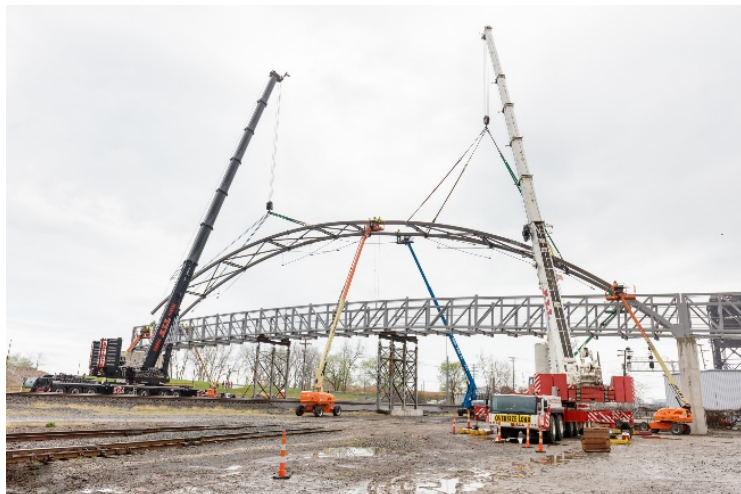
liebherr-all-crane-tandem-hoist-pedestrian-bridge-1.jpg Tandem hoist to place the huge bridge span over the railroad tracks.
