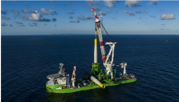
liebherr-deme-orion-installation-monopiles-arcadis-ost-germany.jpg
