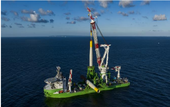
liebherr-deme-orion-installation-monopiles-arcadis-ost-germany.jpg
