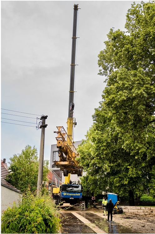
liebherr-ltm1130-5.1-esb-berg-02.jpg Little space - supporting the mobile crane was a challenge.
