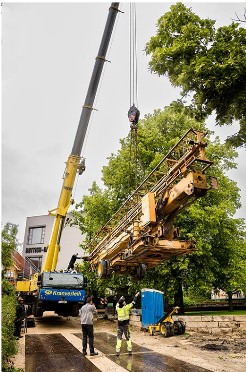
liebherr-ltm1130-5.1-esb-berg-03.jpg Soft landing - the 28 K fast-erecting crane is set down on the site access road for onward transportation.
