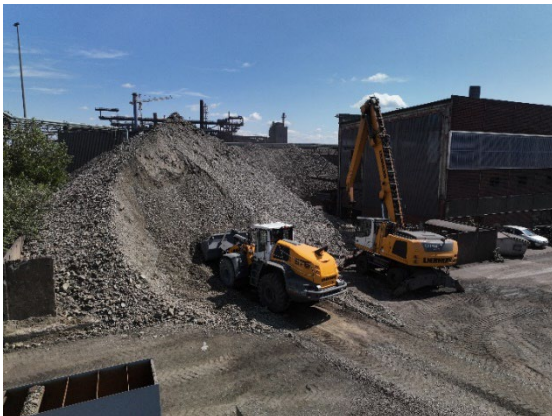
liebherr-earth-moving-machinery-heis-germany.jpg Several Liebherr earthmoving machines are in use at HEIS.
