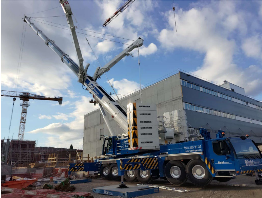
liebherr-ltm-1350-6.1-first-job The Liebherr LTM 1350-6.1 moving concrete columns on its first assignment.
