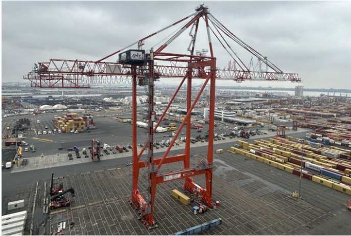
liebherr-pnct-assembled-sts.jpg One of the Liebherr STS as assembly approaches completion
