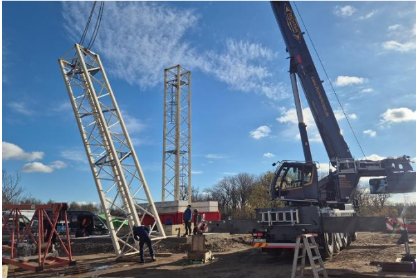
liebherr-ltm-1100-5-3-richter-1.jpg First assignment: the LTM 1100-5.3 assembles a tower crane in Leipzig.
