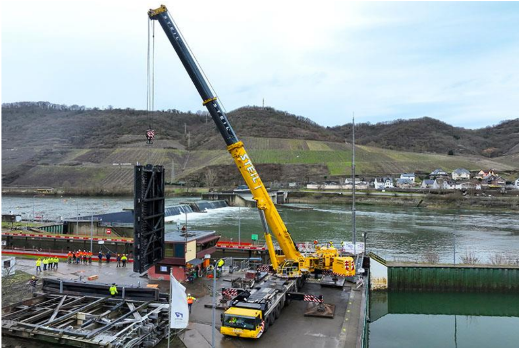
liebherr-ltm1650-9.1-steil-mueden-02.jpg The erected sluice gate is swung into the assembly position.
