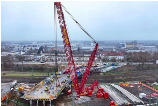
liebherr-lr-1700-1.0-egger-dismantling-bridge
