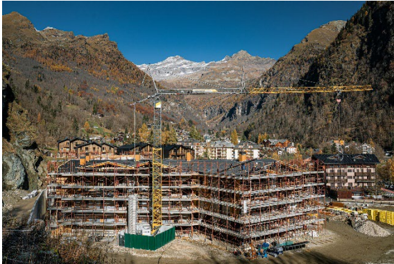
liebherr-81K-cantiere-algna-valsesia-01.jpg Liebherr 81 K building the new mountain lodge in Piedmont.
