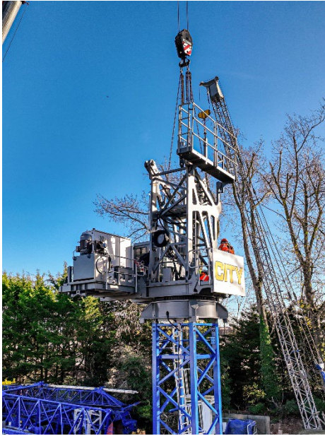
liebherr-uk-city-lifting-195HC-LH-03.jpg The installation of the HMF
