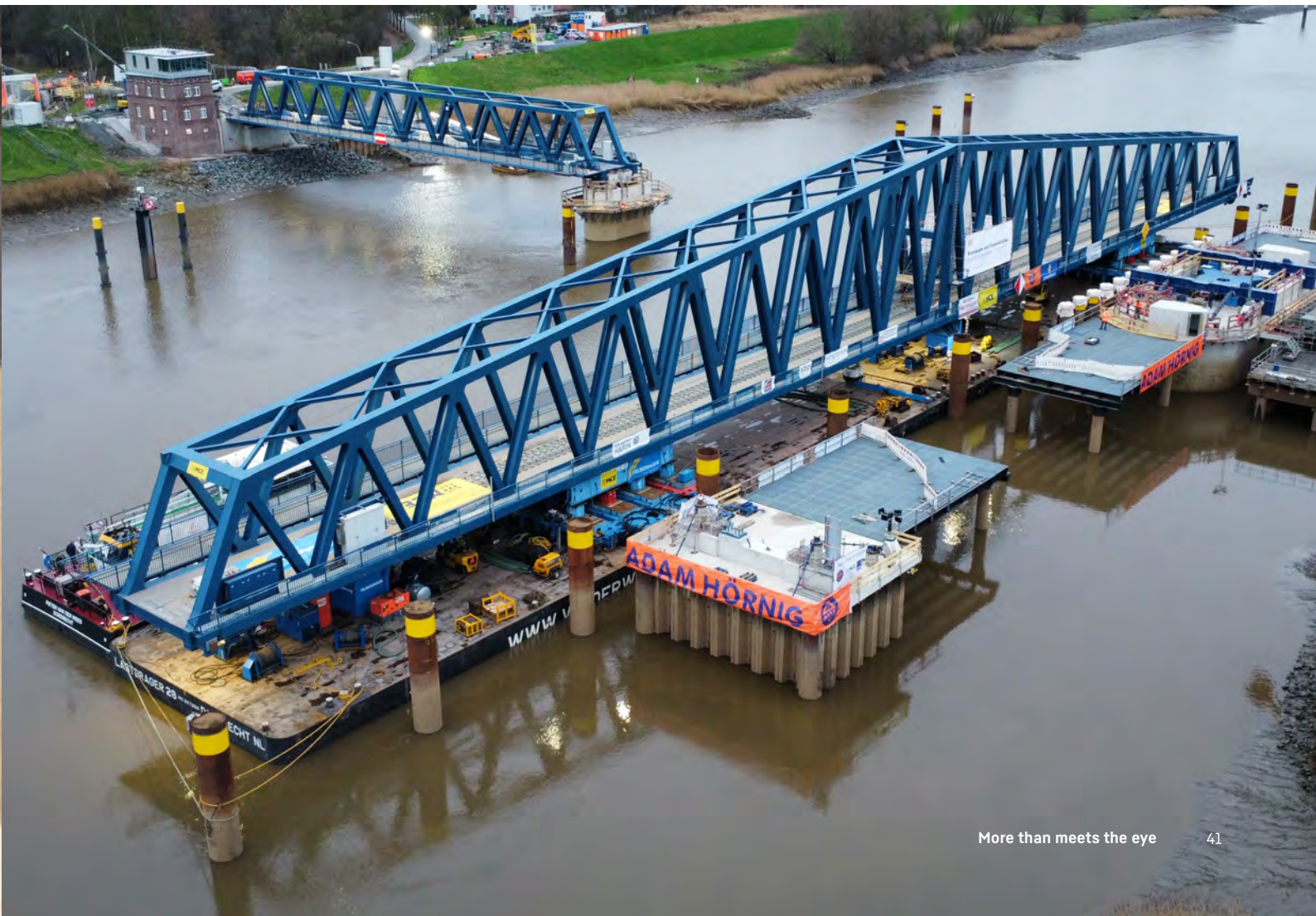
The Friesenbrücke as it's being completed. Image © DB InfraGO AG
