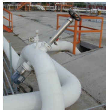
Pipeline installation with quick change fitting
