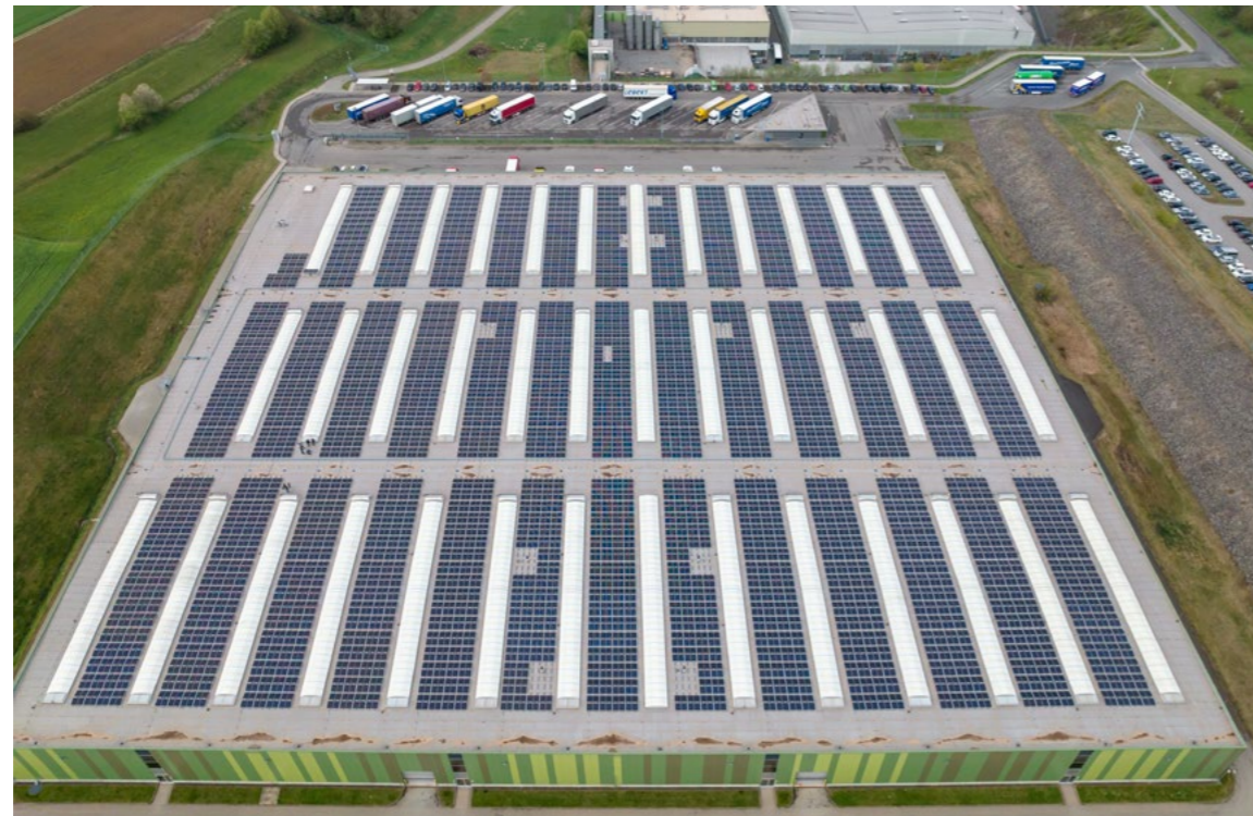
The new 2-MW photovoltaic system in Ochsenhausen
