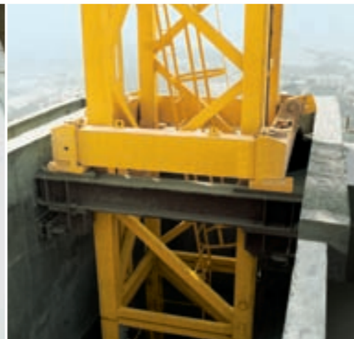
The upper climbing frame of the IC tower.
