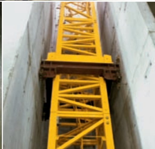
Clamping the IC tower into an elevator shaft.
