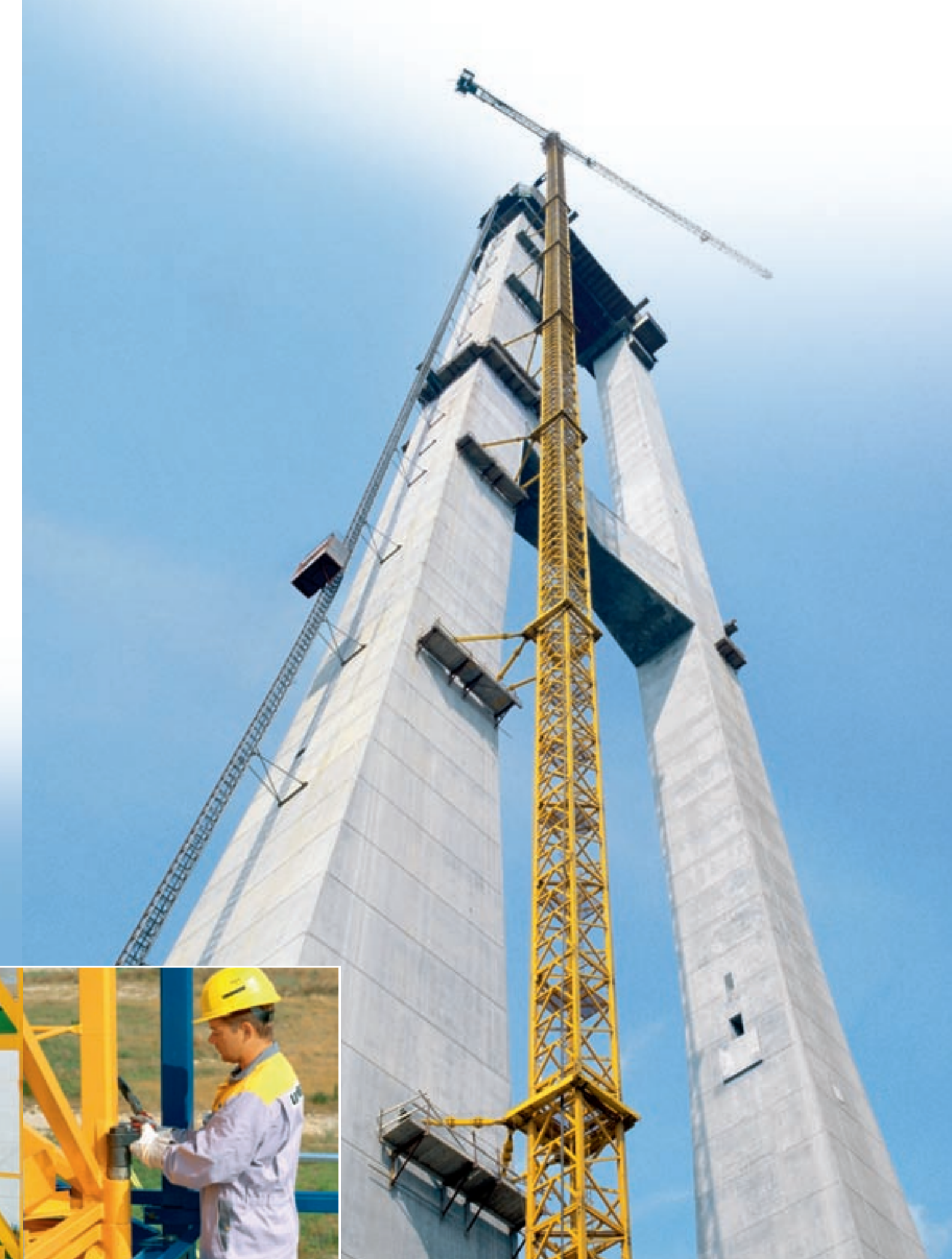
Bolts can be tightened and released quickly using the hydraulic driver.
