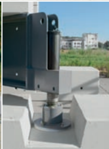
The support spindles for rapid levelling.
