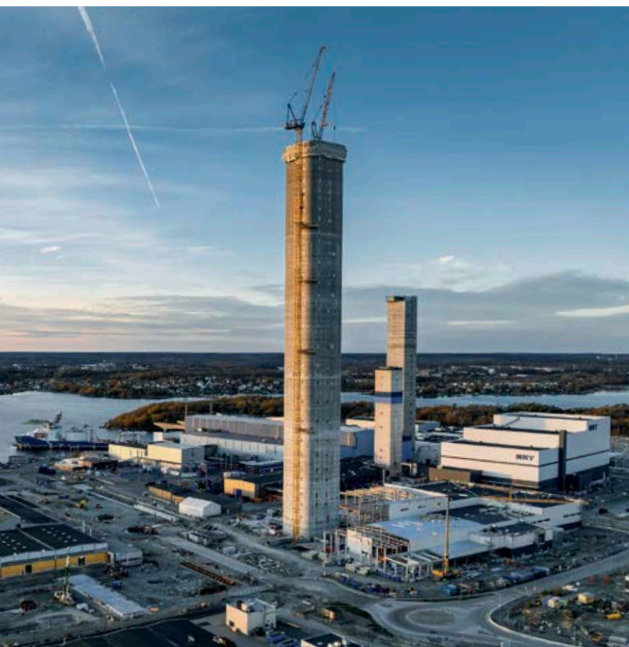
NKT Tower 3 in Karlskrona
