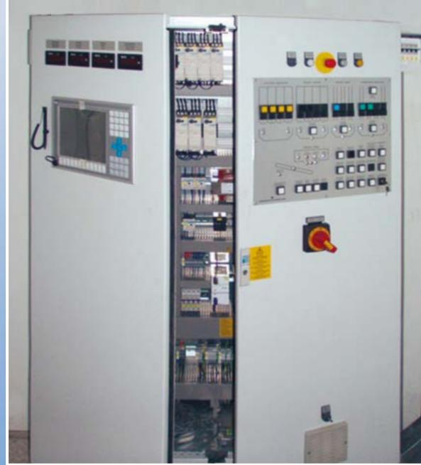
The Litronic-BCS is installed in the switch cabinet to save space.
