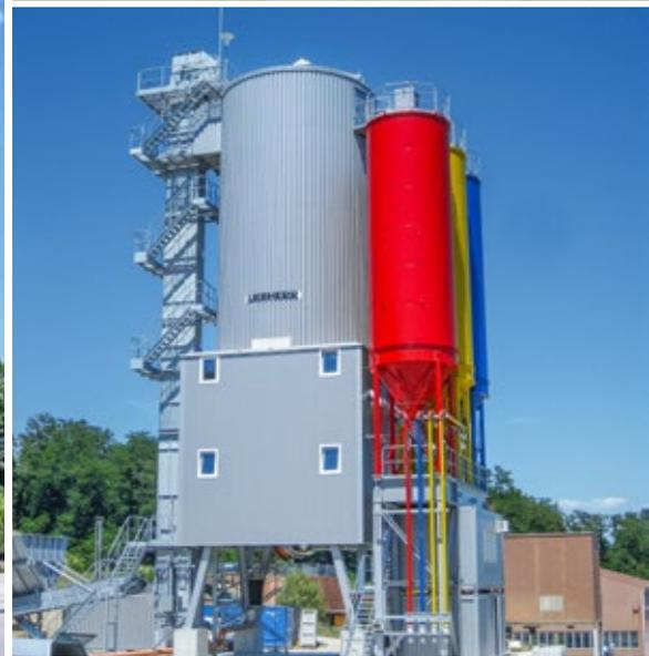
For many years Betomat-type tower plants have been used successfully all over the world for pre-mixed concrete as well as in the prefabricated and pre-cast element production industries.
