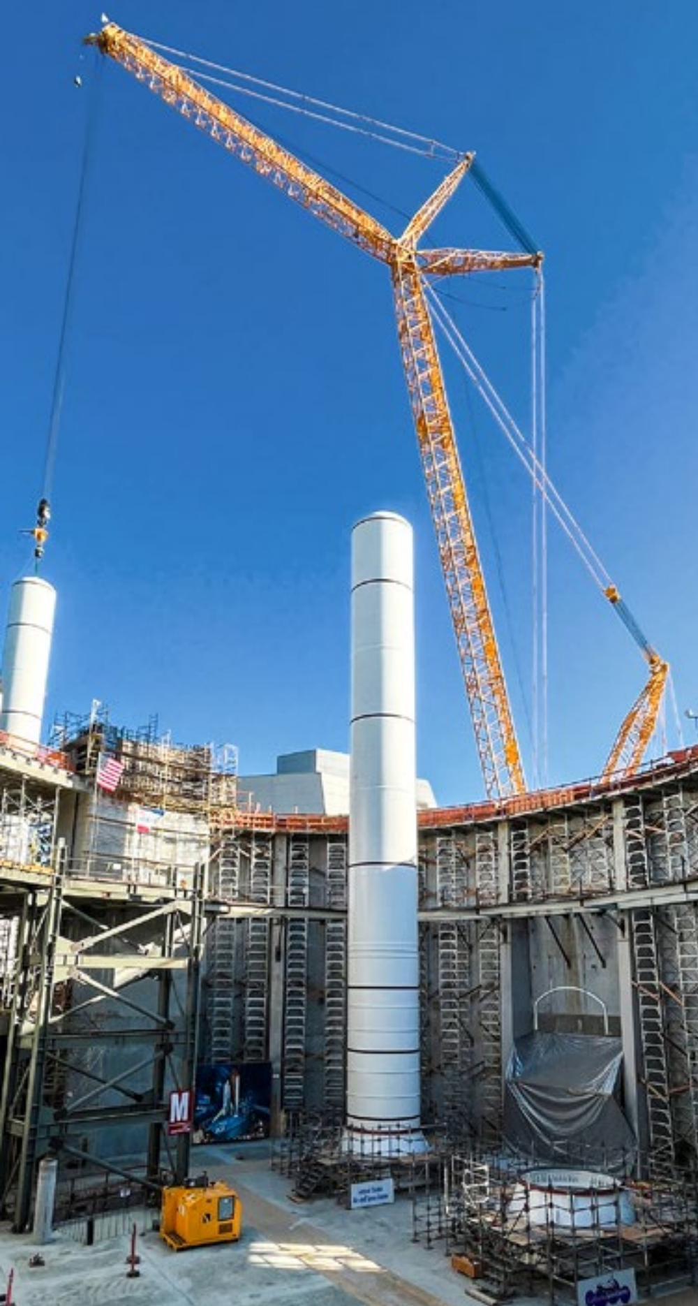
Lift of the solid-fuel rockets onto the mounted aft skirts.
