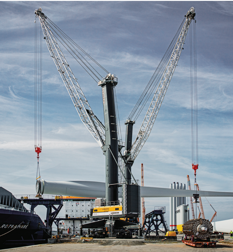
Two Liebherr mobile harbour cranes in tandem lift operation handling rotor blades at the port of Esbjerg (Denmark)
