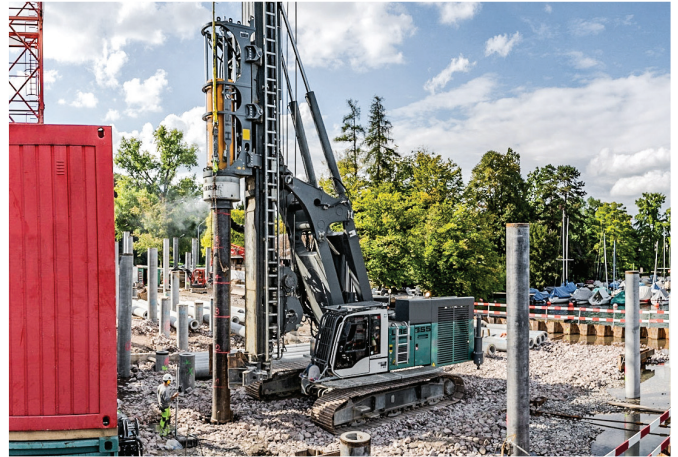
The LRB 355 driving spun piles with the hydraulic hammer H 15-10 at Lake Zurich (Switzerland)
