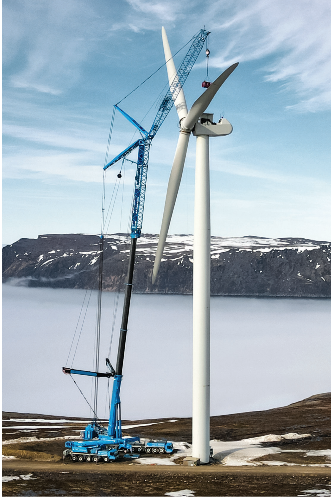
The LTM 1750-9.1 – featuring Y guying, telescopic boom extension and luffing lattice jib – installs a wind turbine in Norway.
